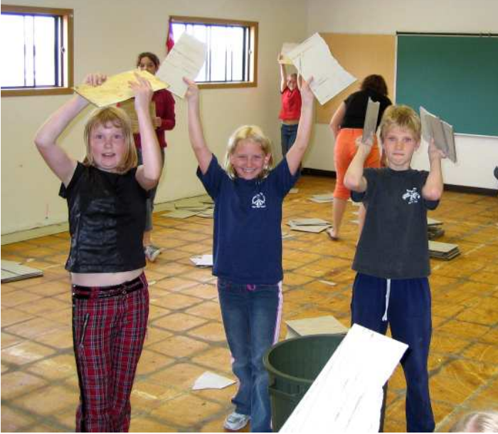
students remove the old tiles in the grade 5/6 classroom
